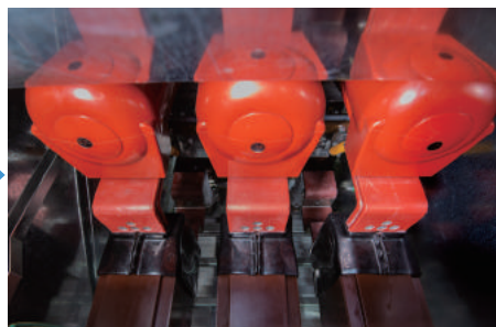
Current transformers are installed in the cable compartment
