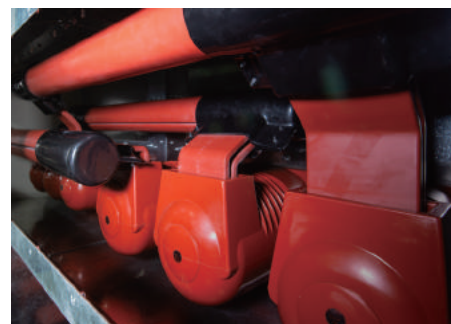
Main busbars (air insulated) with tin plating
