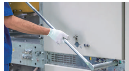
Earthing switch operation
