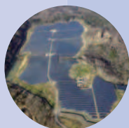
Solar power generation
